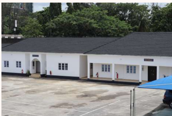
Ariel View of some sections of the renovated office blocks
